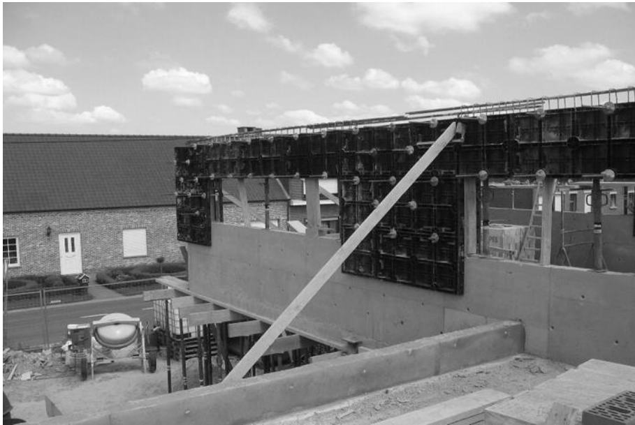
Figure 4: GeoPanel Formwork System in use
